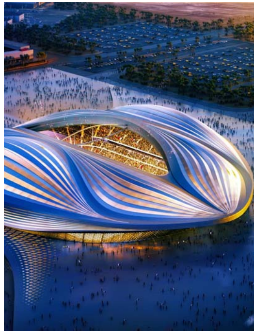
Al Janoub Stadium
