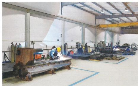
Large Welding Workshop
